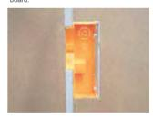
4) Self-drilling screw fastening of the box. Detail of separate space for screw
