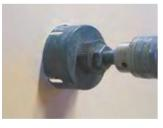
2) Inserting the KUH 1/L box into the prepared hole. Covering the box with the bottom plate.
